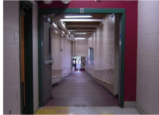
Ramp down to lower gym
