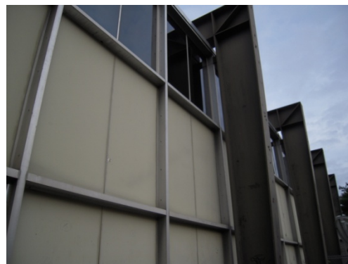
Exposed performance gym structure & curtain wall
