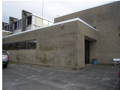
Lower gym entry and ramp to performance gym
